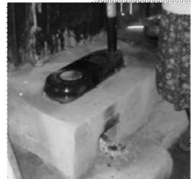
2-pot Chimney clay stove: built using Envirofit Z insert (2,000 ksh) and 2-pot chimney attachment (1,200 ksh); labor est. 400 ksh
